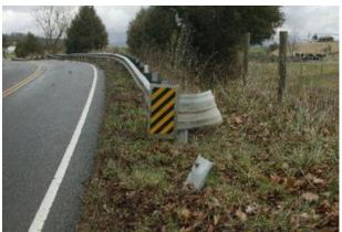
22. Because a "modified ET-Plus's" proper function requires that the guardrail pass through the end terminal, the dimensions of the end terminal components are critical. Even the slightest change to the end terminal can negatively impact the end terminal's ability to function properly and safely for its reasonably anticipated use.
